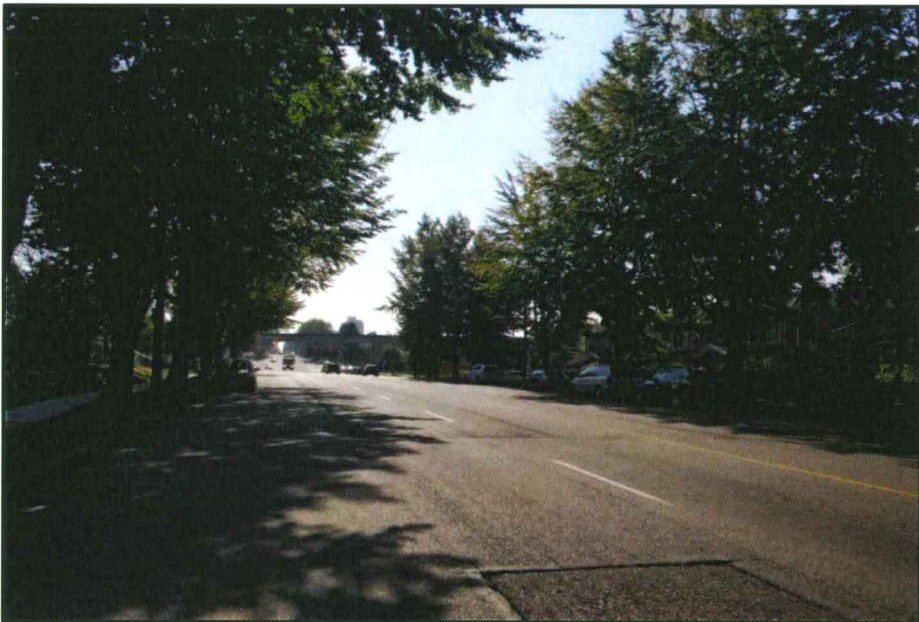
SOUTH VIEW ALONG NANAIMO STREET (SUBJECT PROPERTY TO THE RIGHT)
