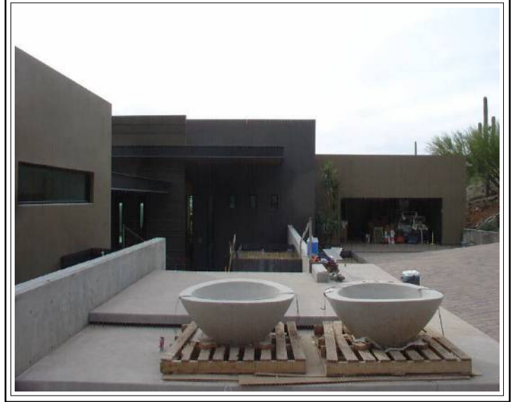
Front subject entry and garage
