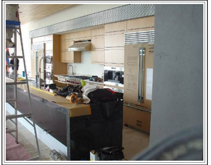
Secondary kitchen view
