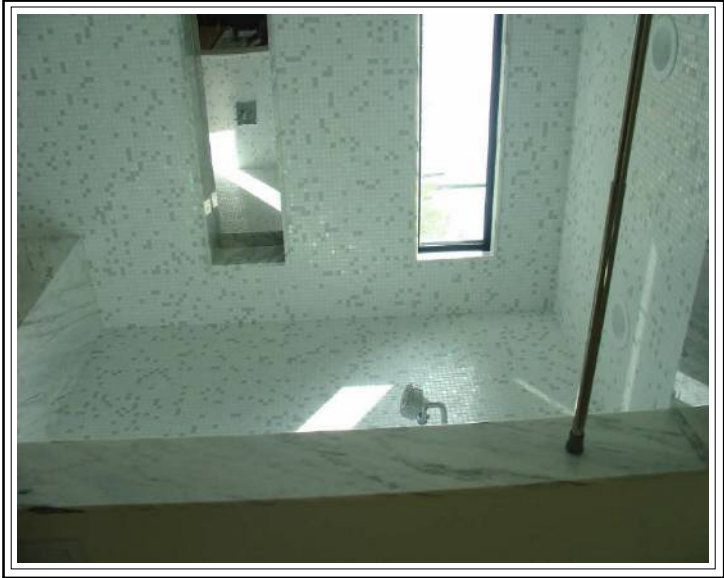
Bathroom tile shower detail
