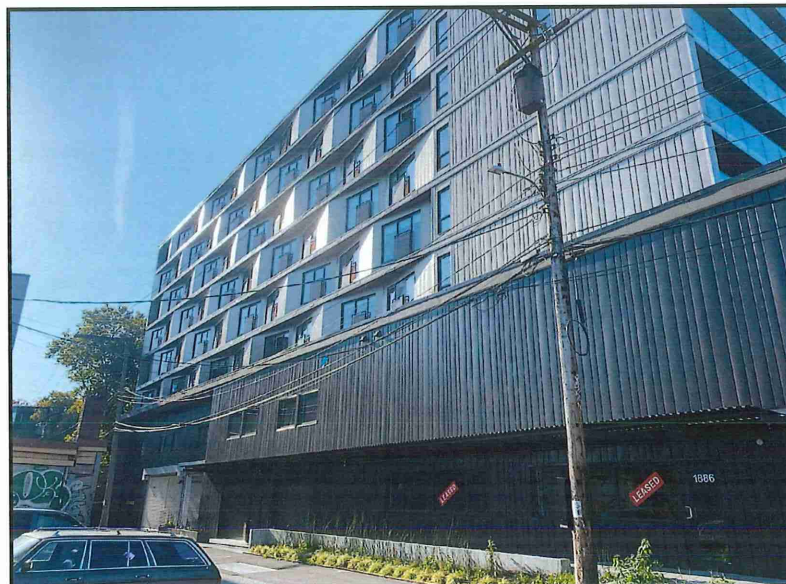
LOOKING SOUTHEAST FROM INTERSECTION OF REAR LANE AND SCOTIA STREET
