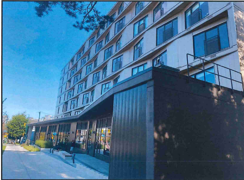
LOOKING NORTHWEST ALONG THE E 2 ND AVENUE FRONTAGE
