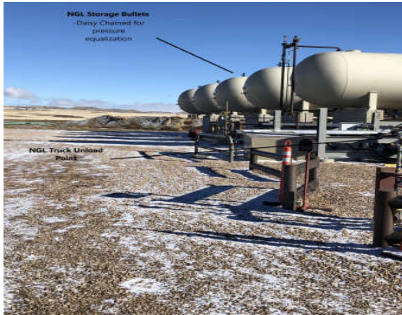
Figure A-6: The daisy-chained NGL storage bullets
