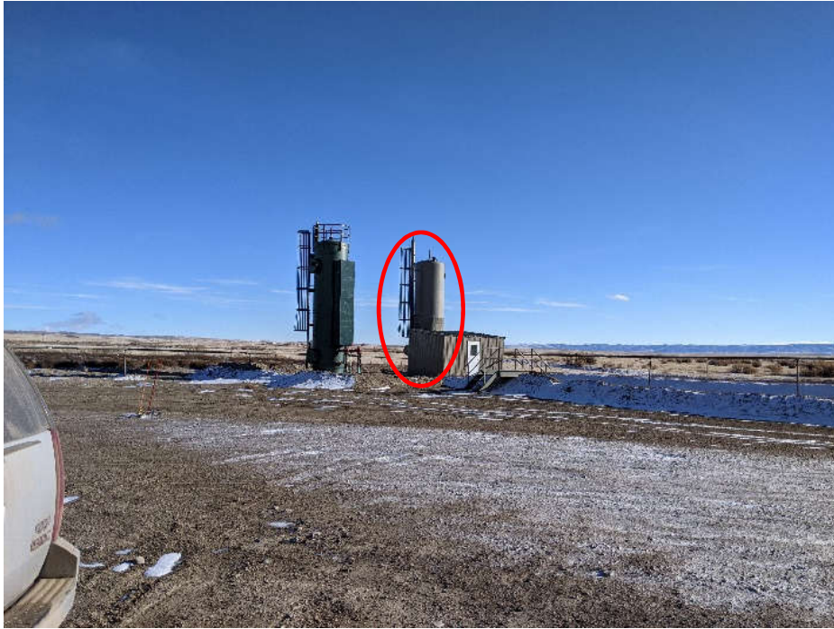
Figure A-2: Example of a single well battery heater-treater unit, circled in red
