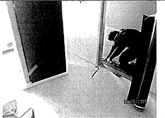
Installing Laminate Flooring on 4<sup>th</sup> Floor
