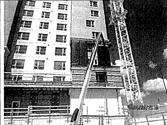
Prepping for Cement Panel on South Elevation
