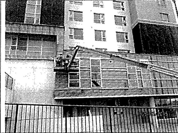
Installing Rain Screen System at North Elevation
