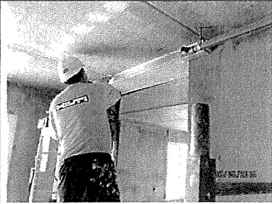
Provide Fire Rating Steel Lintel on 12<sup>th</sup> Floor
